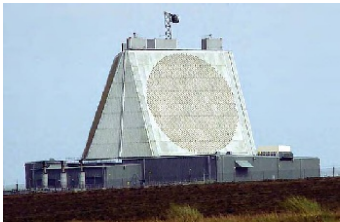
The Solid State Phased Array (SSPAR) at RAF Fylingdales, UK. (Image: wikipedia.org)
